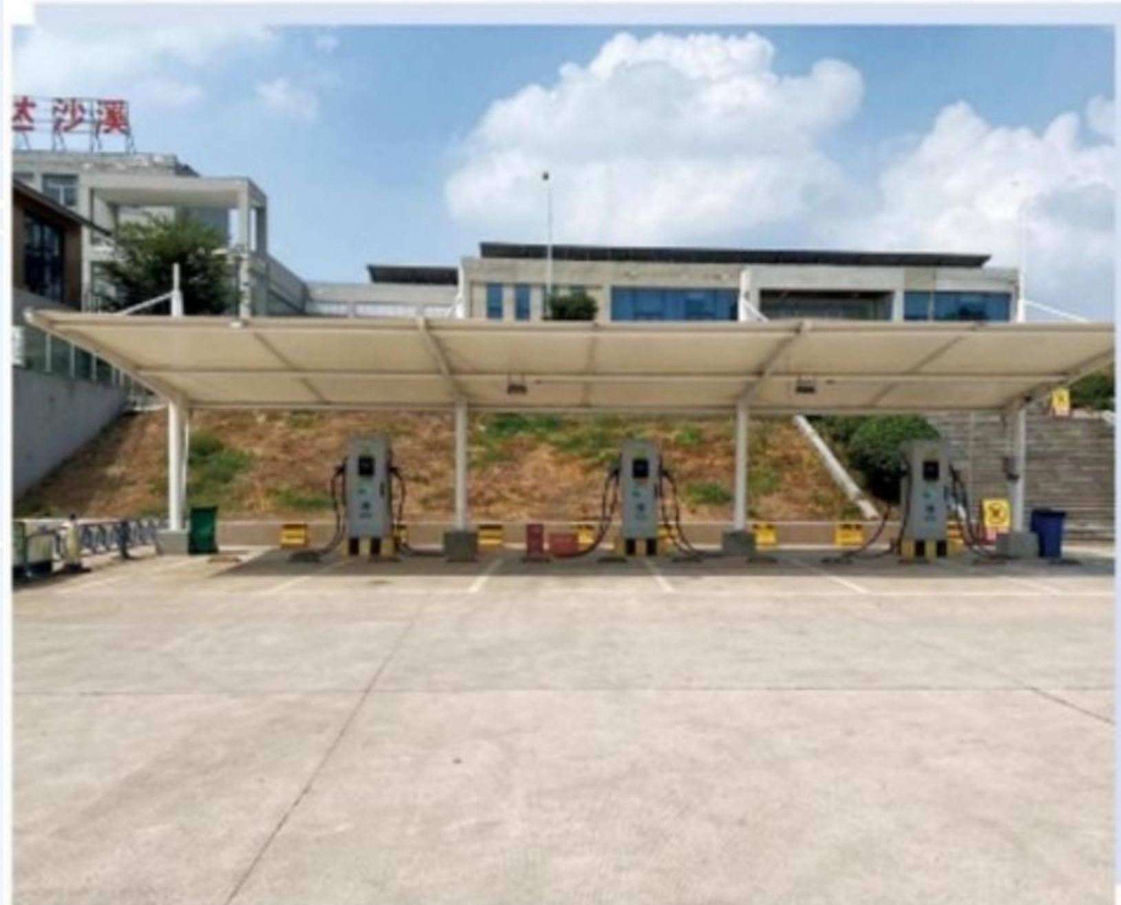
Shaxi Service Area on the Jing-Tai Expressway
