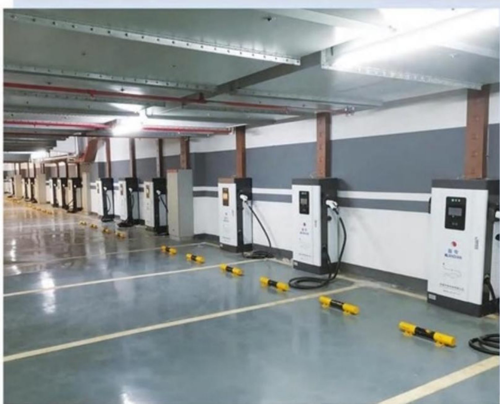
Zhejiang Liandu Building
