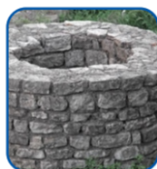
Well Water Boosting
